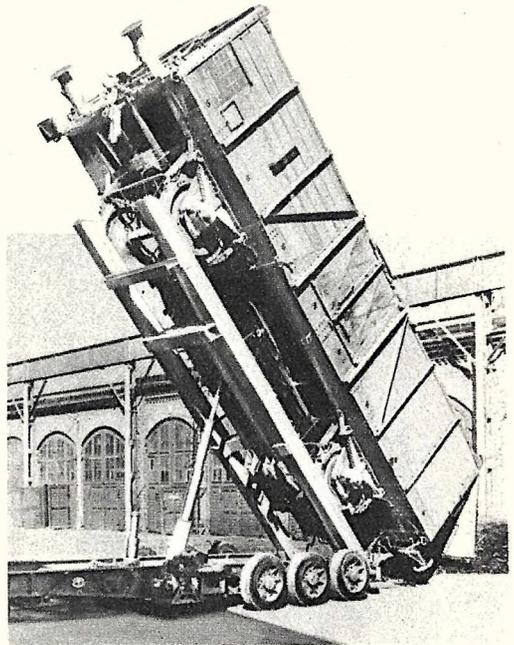
This specially designed trailer truck now in use by German railways delivers rail shipments to remote places where service is not available. A hydraulic lift tilts car for unloading.
