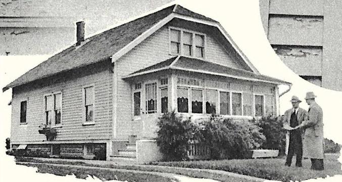
The house at the left was built in 1931 and painted with pure white lead, a satisfactory job. In 1934 it was repainted with a hard, quick-drying paint. The above photograph was taken only a year after it was applied.
