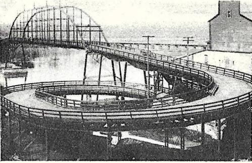
This Minnesota bridge, built high over the Mississippi to give river steamers enough head-room, has an approach ramp that spirals groundward to permit automobile vehicular traffic.
