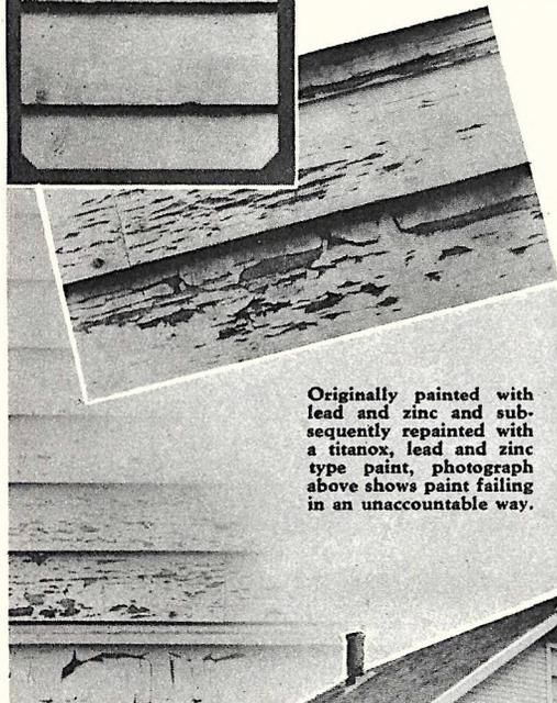
Originally painted with lead and zinc and subsequently repainted with a titanox, lead and zinc type paint, photograph above shows paint failing in an unaccountable way.
