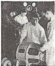
Checking motor windings in Electrical Department.
