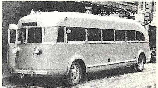
Featuring a body constructed of aluminum instead of the usual steel, this modern bus reduces gross weight by two tons. A V-8 Ford motor is sufficient to power the new motor coach.
