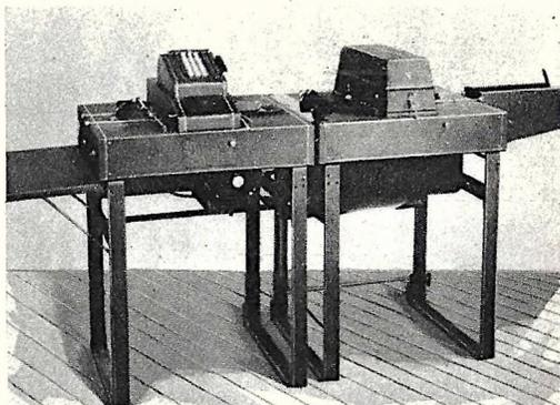
This electric protectograph working in tandem with the check signer on the right can turn out 2,500 checks, written, signed, and numerically stacked in an hour. They also operate singly.
