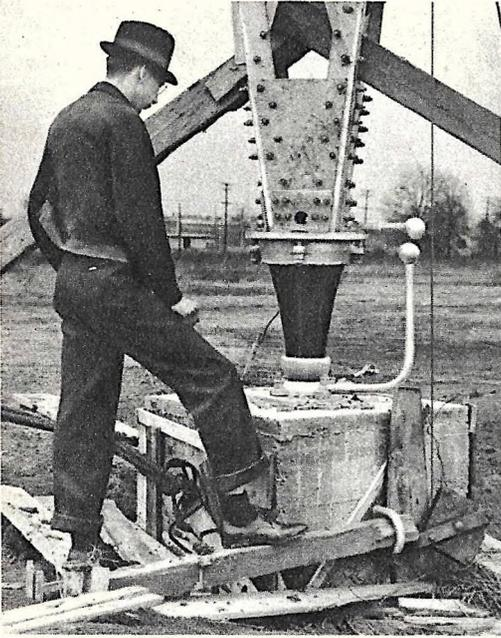
This porcelain base supports an iron radio tower reaching 390 feet into the air. The base is 6 inches in diameter and only 18 inches long. Total pressure on porcelain base is 120 tons.
