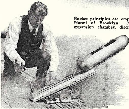
Nanni here demonstrates how his 10 passenger, steel lifeboat will be launched. Rubber cushions will reduce starting and landing shock. The boat cannot turn or twist in the air.
