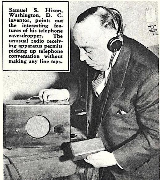
Samuel S. Hixon, Washington, D. C. inventor, points out the interesting features of his telephone eavesdropper. The unusual radio receiving apparatus permits picking up telephone conversation without making any line taps.
