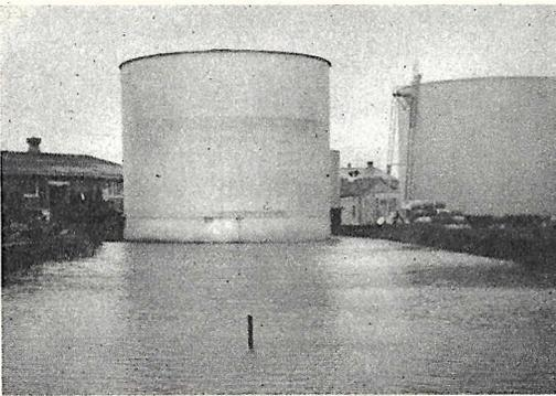
This new tank with a capacity of 330,000 tons was literally floated to a new site. Engineers erected an earthen dyke, filled it with water then towed the tank to its destination.
