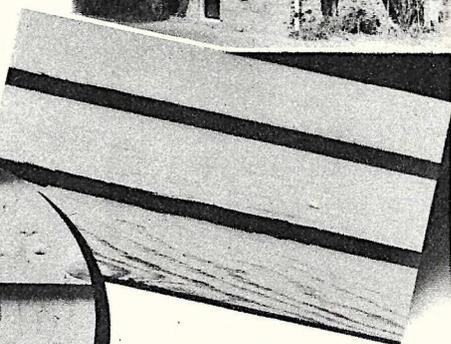
The house up above was not painted for eight years. From a distance the paint looked shabby. A closeup photo reveals the paint worn down to bare wood. Two new coats will fix it up fine.
