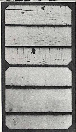
On three sides of the house pictured here, the paint cracked and scaled badly—see left photo. On the fourth side, the side fully exposed to weather, paint gave excellent service, as shown in lower left photo. On the bad sides the wood carried six coats of paint, the good side only three.
