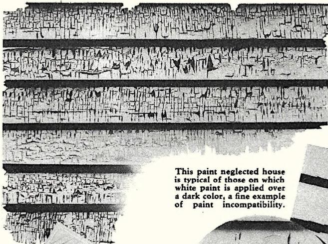
This paint neglected house is typical of those on which white paint is applied over a dark color, a fine example of paint incompatibility.
