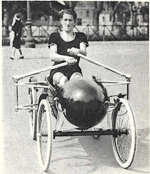
Bringing the features of scull racing to dry land is made possible with this land canoe, the invention of an Italian. Vehicle is propelled by oars which actuate a gear mechanism.
