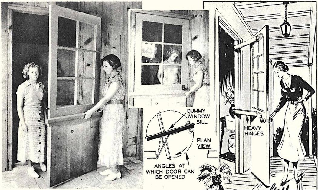
In order to preserve the symmetry of the outside of the home one constructor struck on the idea of a door patterned after the windows. Special hinges were provided so as to permit the door to swing out from the wall and provide an additional exit. The above photographs and drawing show how this type of construction might be applied to other types of dwellings.
