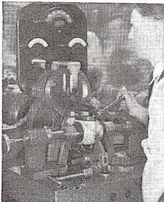
*This special testing machine checks the distributor for timing, automatic advance, and vacuum brake setting.*
