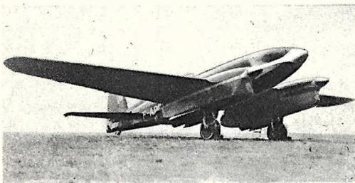
Here is the secretly built French plane which hopes to span the Atlantic in 40 hours and return. Powered with Renault motors, the ship has a cruising speed of 200 miles an hour.
