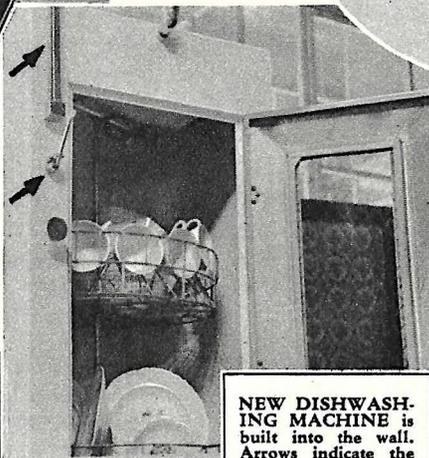
**NEW DISHWASHING MACHINE** is built into the wall. Arrows indicate the mechanism which injects cleansing chemicals into the water.
