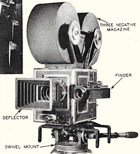
Here is a front view of the three-color Technicolor camera. In the magazine are three negatives side by side. One negative records red-orange, another blue-green, the third, yellow. A prism behind the single lens divides light rays into colors.
