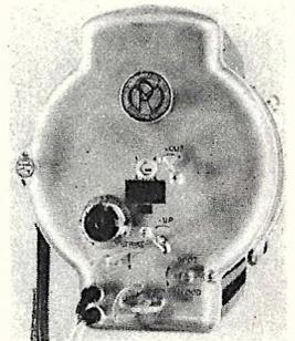
Above—The controls of the sun-arc can focus the light on such a small spot it will ignite wood. The numerous controls are essential for accurate lighting. Left—Two men can handle the sun-arc while on earlier models six were required. The lens screens out ultra-violet rays and is similar to those which are used in lighthouses.
