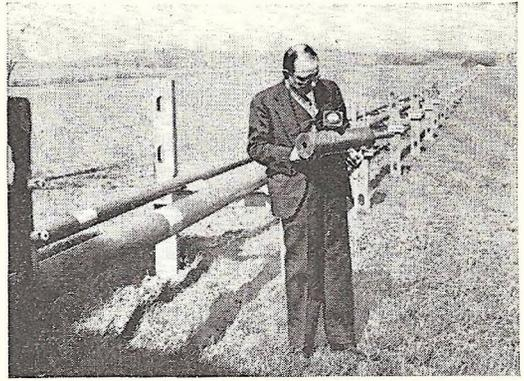
Dr. George C. Southworth is shown here inspecting his pipe-line system for conducting ultra-high frequency radio waves. Waves pass through pipes like sound through a speaking tube.
